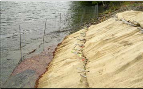
Riparian demonstration project following planting, Spring 2005
