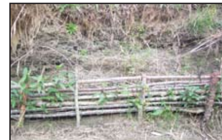
An example of a bank stabilization project.
